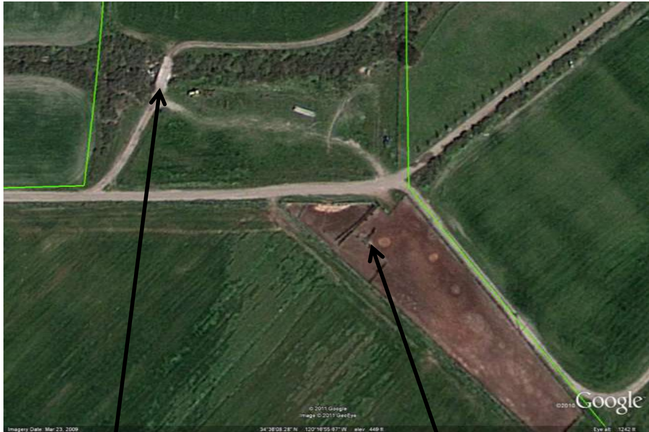
Entrance into Well Field
